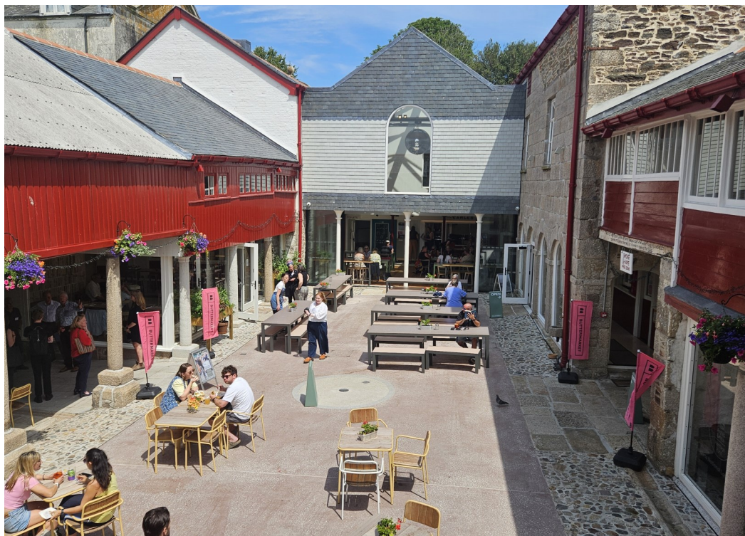
The Courtyard at the Buttermarket in Redruth, Cornwall, which was completed and re-opened in 2024/25.
