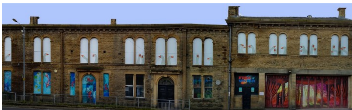
Sowerby Bridge, West Yorkshire, before works. Fire and Water
