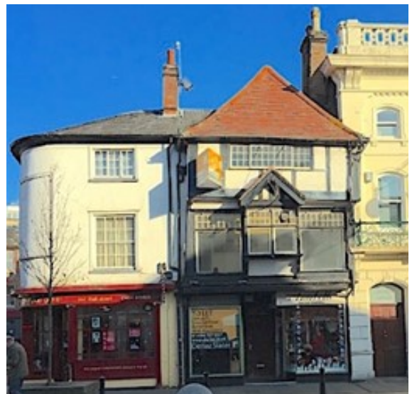
2-3 High Street, High Wycombe, before works. Buckinghamshire Historic Buildings Trust
