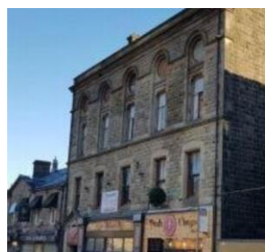
Ramsbottom Co-op Hall Heritage Trust Ltd
