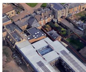
Light Project Peterborough
