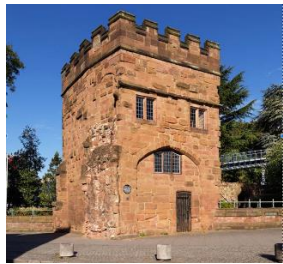
Historic Coventry Trust City Gates, Hales Street, Coventry, West Midlands
