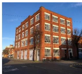
Generator Loughborough CIC
